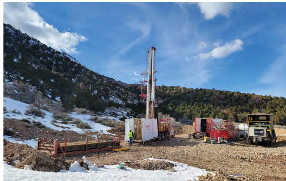
Surface exploration drilling at the Deer Trail Project.
