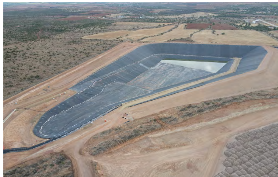
Tailings storage facility under construction at the Juanicipio Project.
