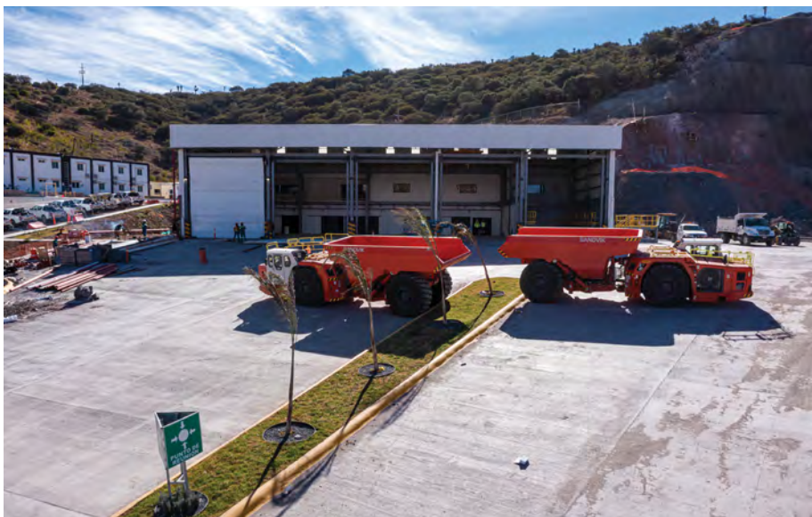
Regular maintenance of the mining fleet is part of the energy efficiency program at the Juanicipio Project.
